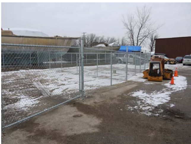
New fencing installed
