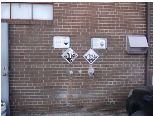
Filling lines before construction
