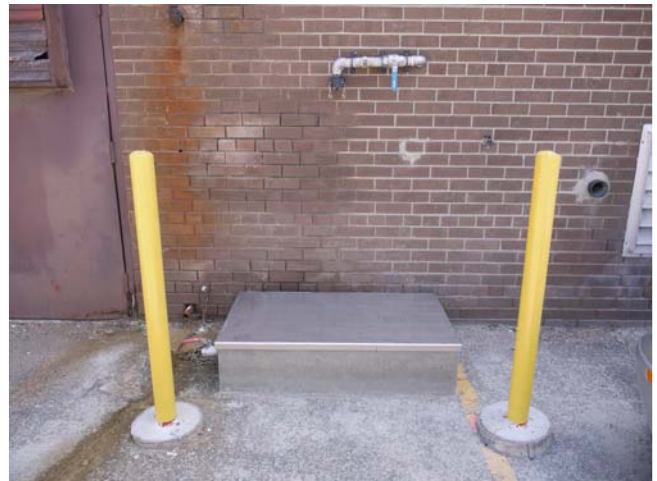
Filling lines after construction of spill containment sumps and bollards
