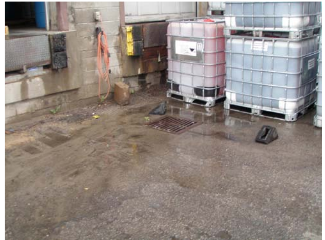
Catch basin in close proximity to loading dock
