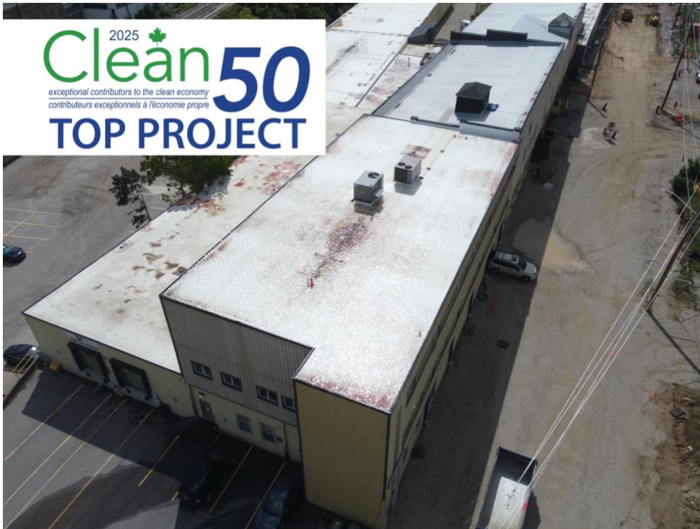
An aerial view of Enviro-Stewards’ award-winning blue roof in action.
