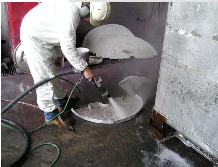
Employee using soluble media blasting
